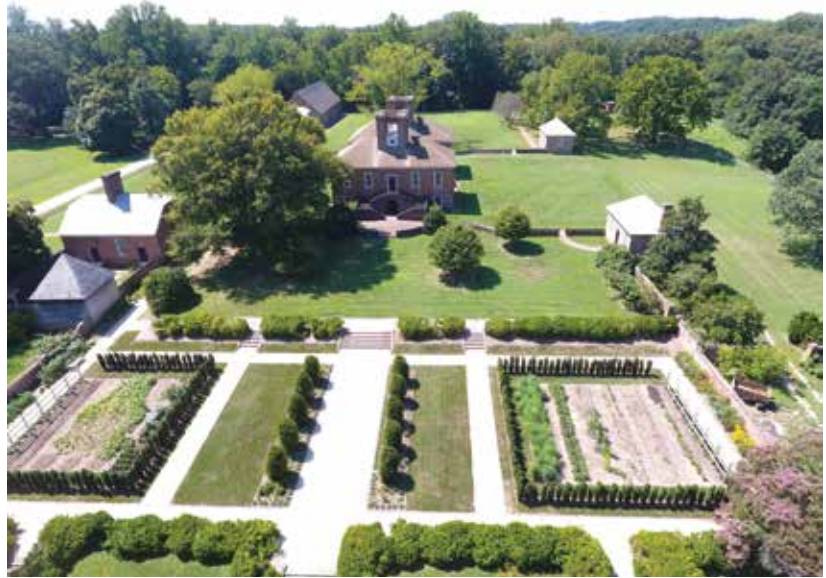
Aerial shot of the Stratford Hall GCV garden restoration. Photo by Matt Peterschmidt
